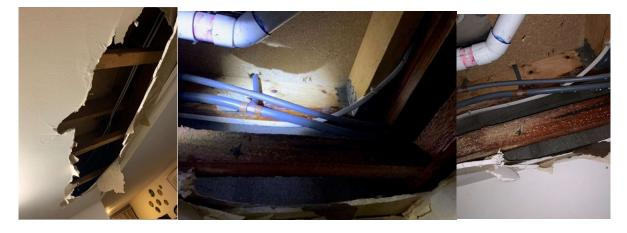
We have got three units leaking through kitchen ceiling about ensuite shower leak and one case with T connection broken above the kitchen ceiling causing whole ceiling cashed.
