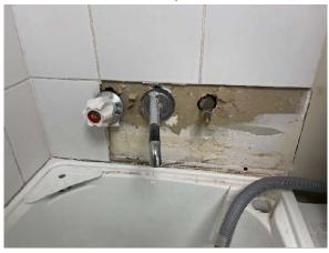
5. Silicon missing behind the taps, water flows along the tile wall getting behind taps and gets to kitchen ceiling above the fridge area.
