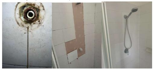
4. Seats crack in laundry tap, it cost \$300 to remove two tiles and change seat and to join behind the wall, to put tiles back on.
