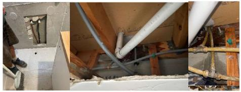
Leak behind the shower tap wall where the copper join is, you are looking around \$1200 to replace all old pipes, remove the sheet and replace with shower mixer and divider for bath. Resheet, water proof and put on new tiles. The cost does not include plastering and painting.
